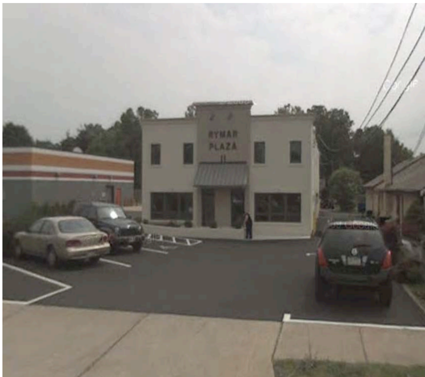
FRONT AND PARKING LOT
